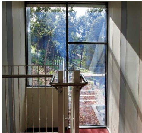
Figure 2. Example of haze (Viridian Glass, 2025)
