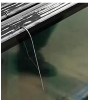
Capillary tube in double glazed unit
