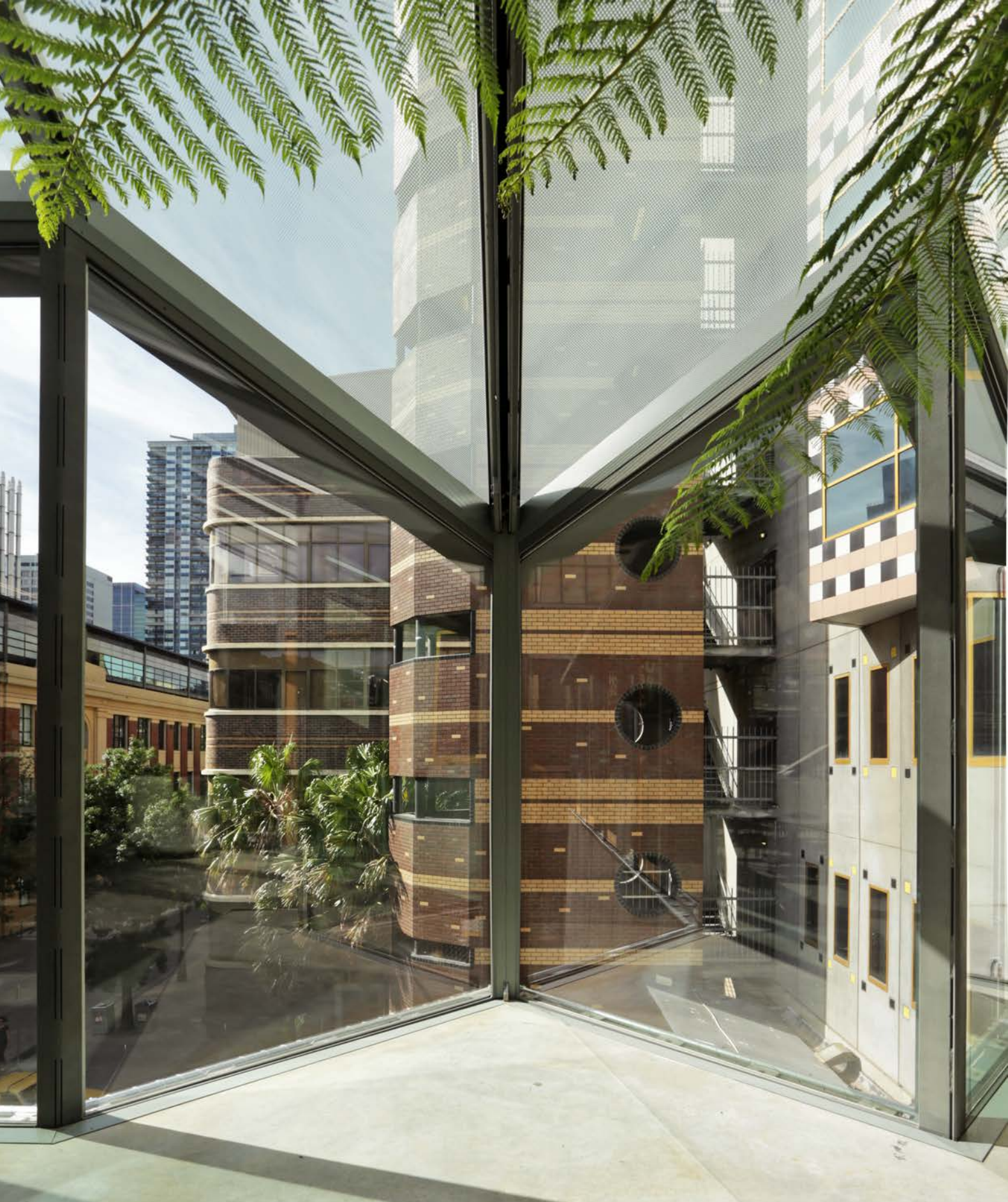
The new Garden Building and terrace at the rear of Building 8 is especially open to its location and adjacent upgrades. Roof glazing is Viridian ScalaSeraphic™ – a product used extensively in the whole re-development to assist with mediation of direct sunlight.
