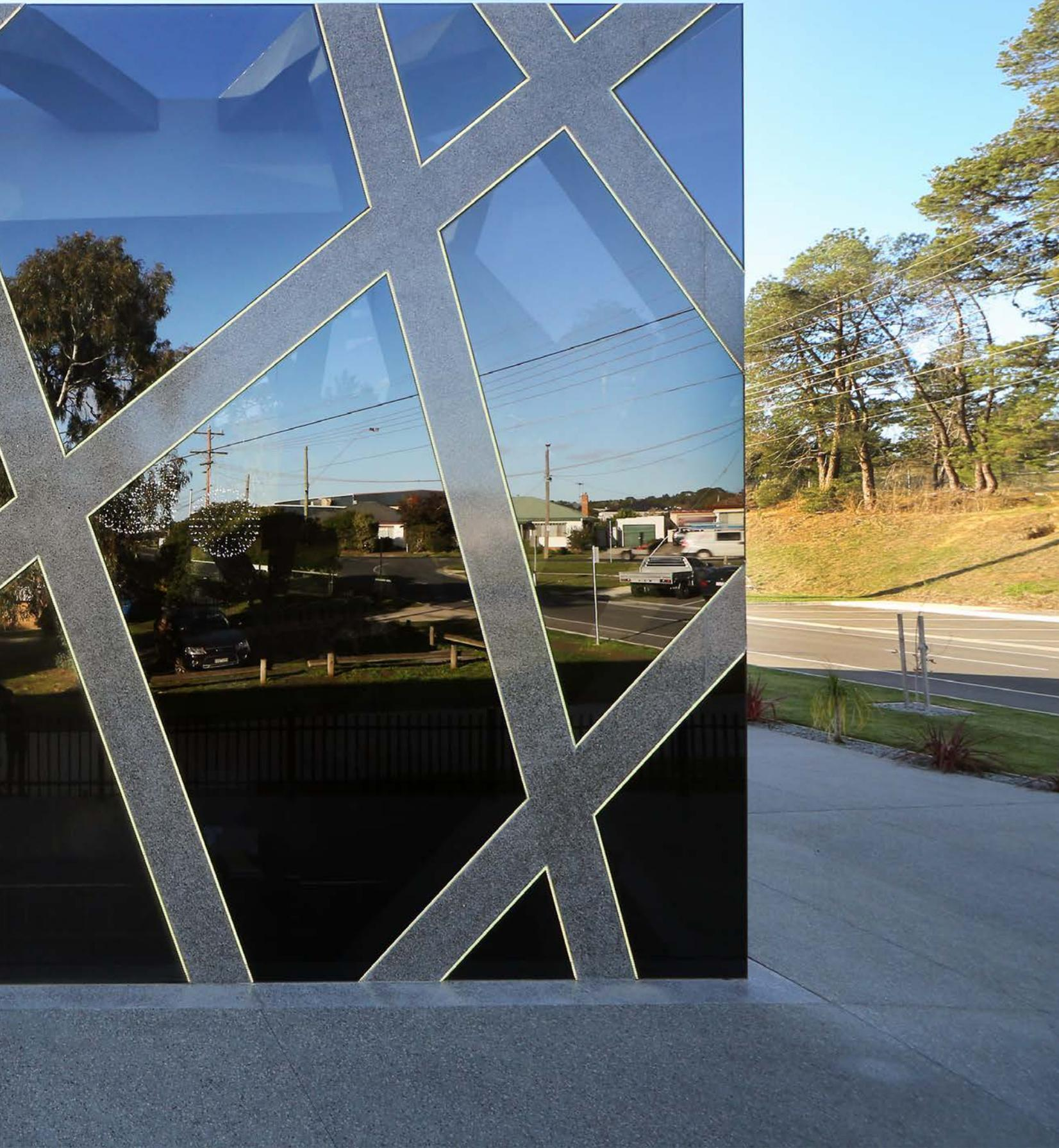
A series of individual laser measured 'window' gaps required millimetre perfect fit with bespoke Viridian glazing.
