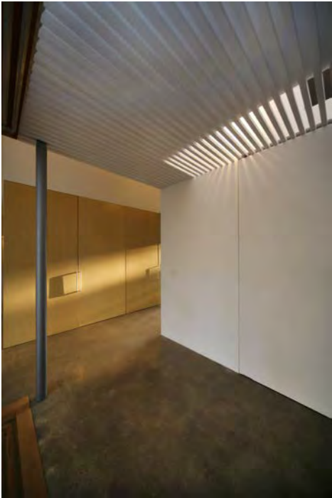
Simple techniques of bringing daylight deep within include central skylights and streamlined detailing.
