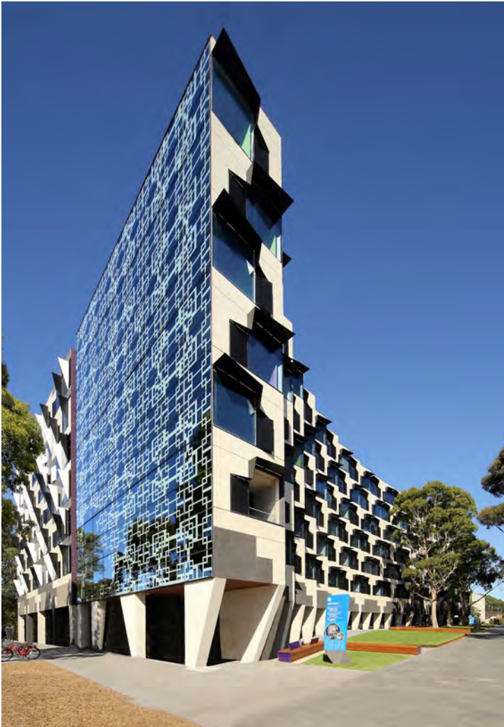
Previous page, left and above: The dramatic north and north-east elevation of Logan Hall with soon to be installed retail spaces planned for the building's undercroft.
