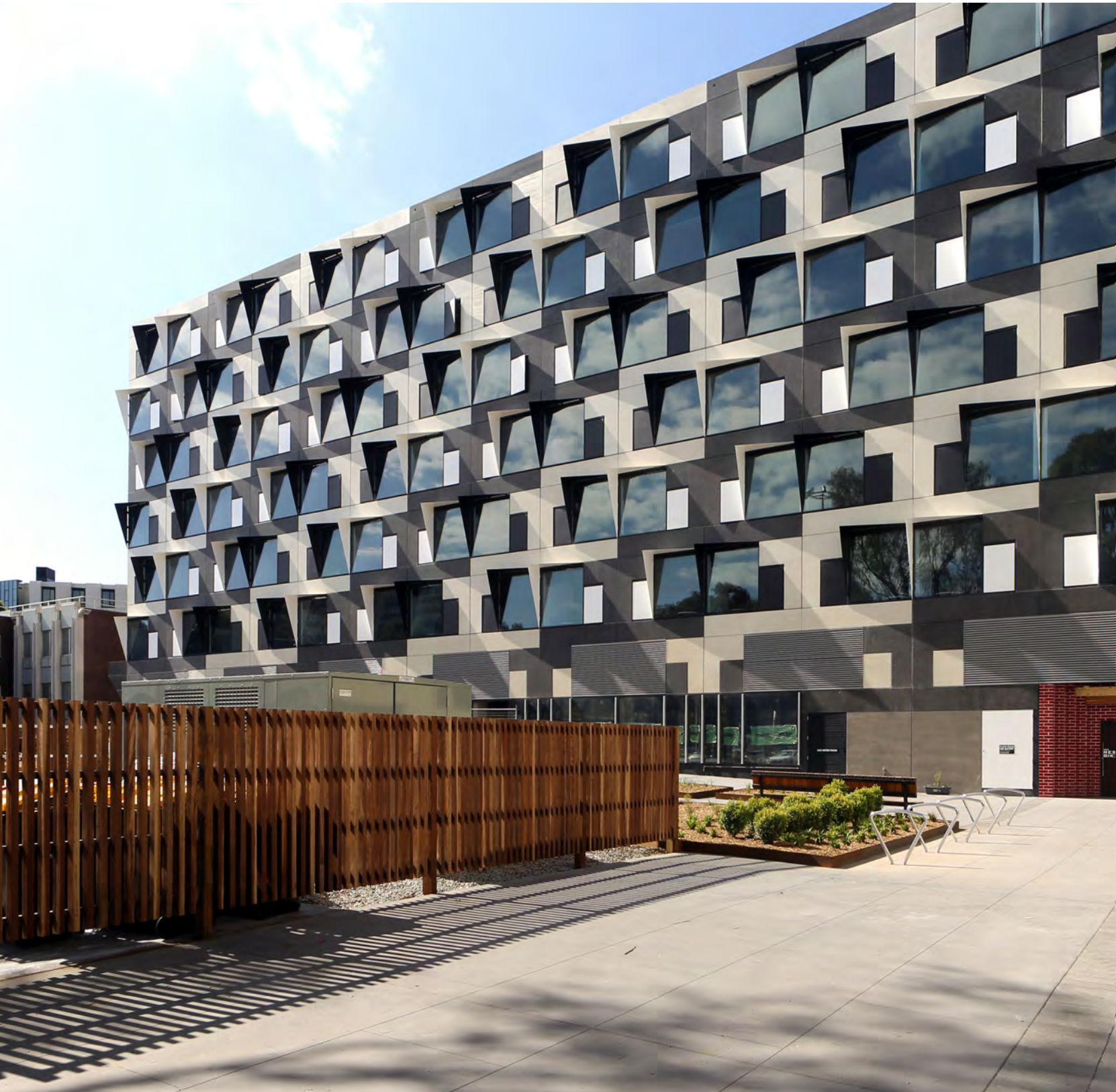
A chequer-board of glazing, triangulated window hoods and reflective glazing richly animate the south-west elevation and courtyard of Logan Hall.
