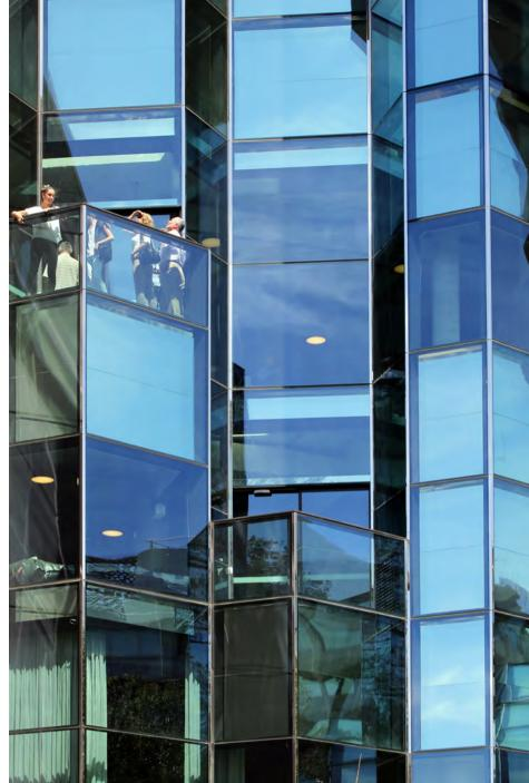
The glazing has a very crystalline, jewel-esque quality. That's highlighted by the polished stainless steel on the leading edge of the glazing.
