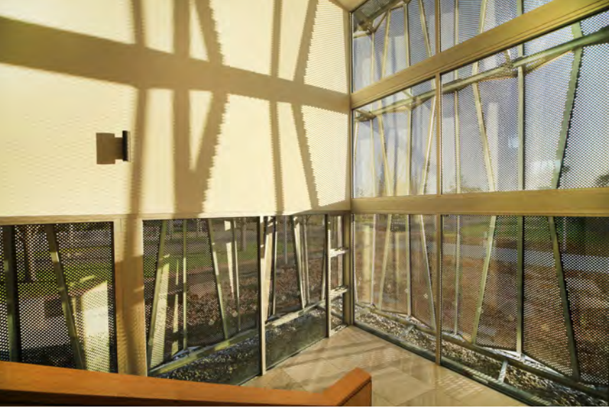
Perforated metal screen and large sheets of VFloat™ usher veiled light into the main foyer/staircase. Two central performance spaces.
