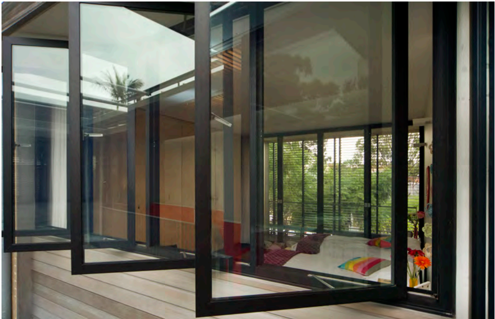
Pivot glazing to courtyard of both bedrooms. Right: Leafy fringe and screened front of house as springboard for community connection.
