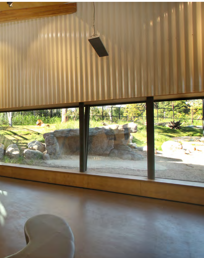
The education and observation centre grows from the composite structure of lightweight, laminated timbers, steel and Viridian glazing to provide a virtually uninterrupted vista.
