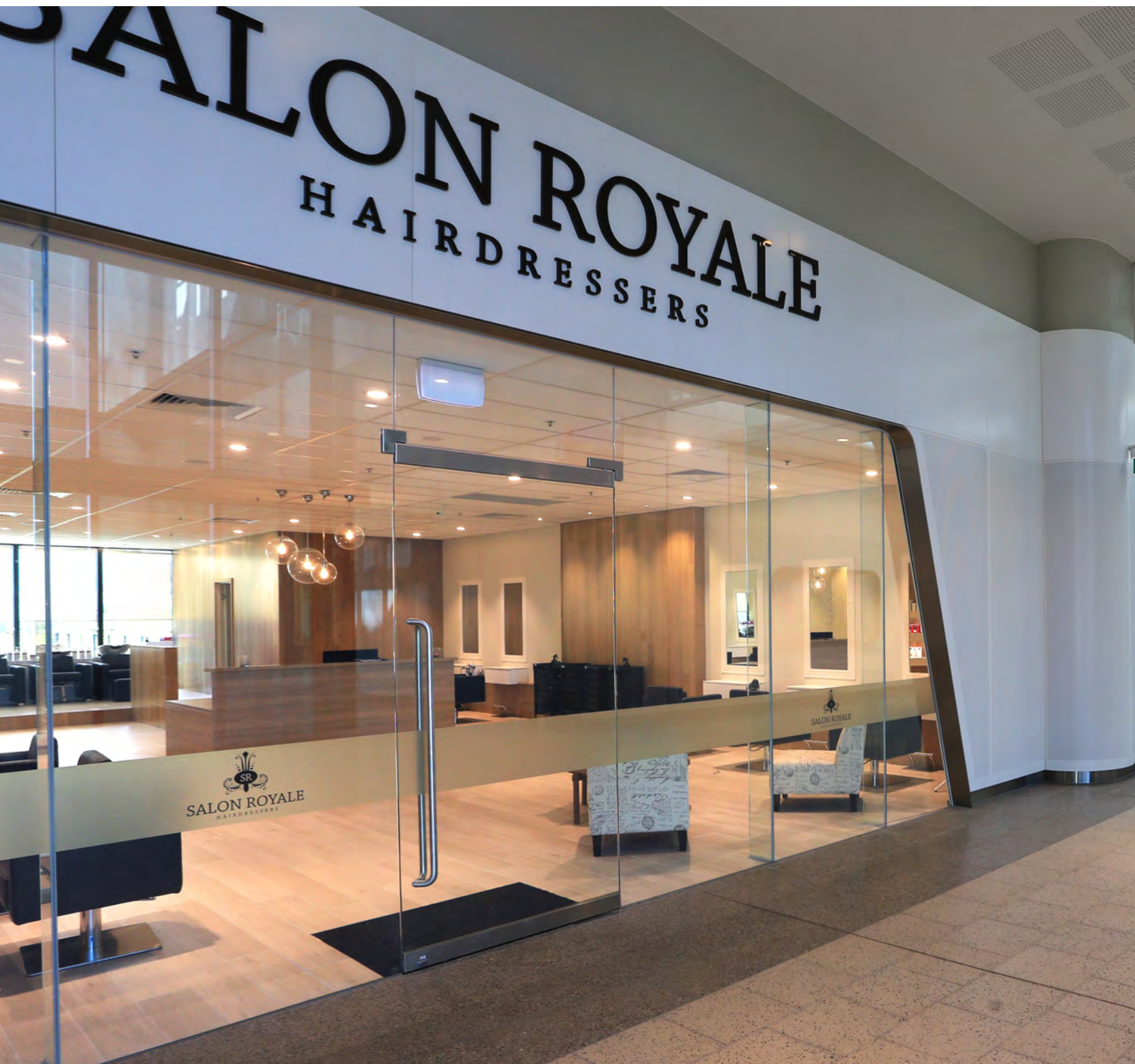
The new, commercial avenue connecting to the hospital has a series of new high-visibility Viridian glazed shop-fronts.
