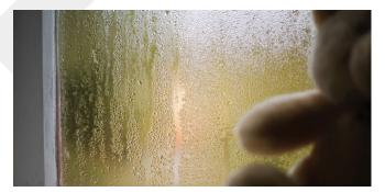
In summary, condensation is a climatic condition that is caused by water vapor changing back into a water form. Glass does not cause the condition, therefore it is not considered to be a product fault.
