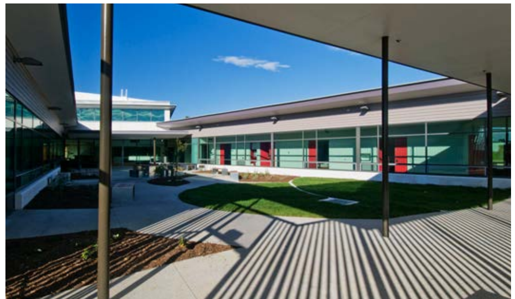
Project: Canberra Hospital Adult Mental Health Facility. Photographer: Brian Steele.
